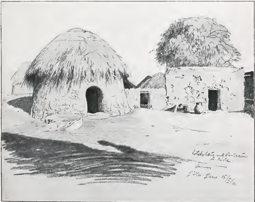
137. Kotoko house in Gulfei with washhouse and kitchen.
